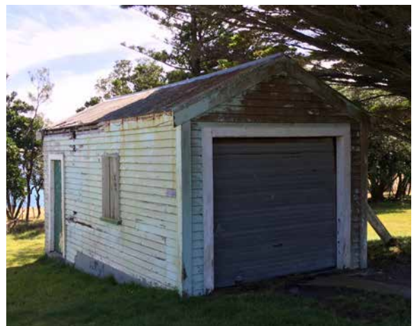
The Lightkeeper's garage.
