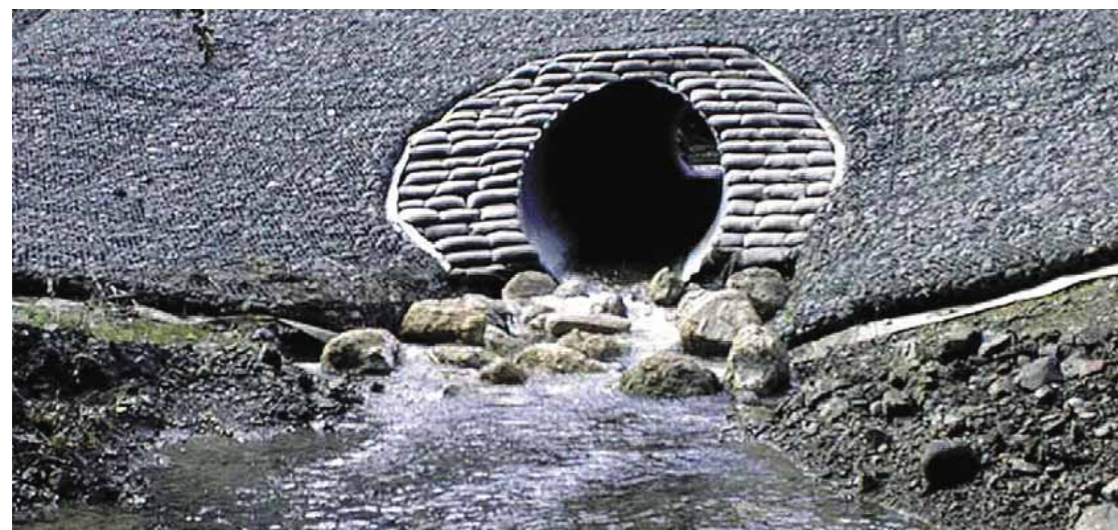
Sandbags and rock placed around the outlet of this culvert help prevent erosion
