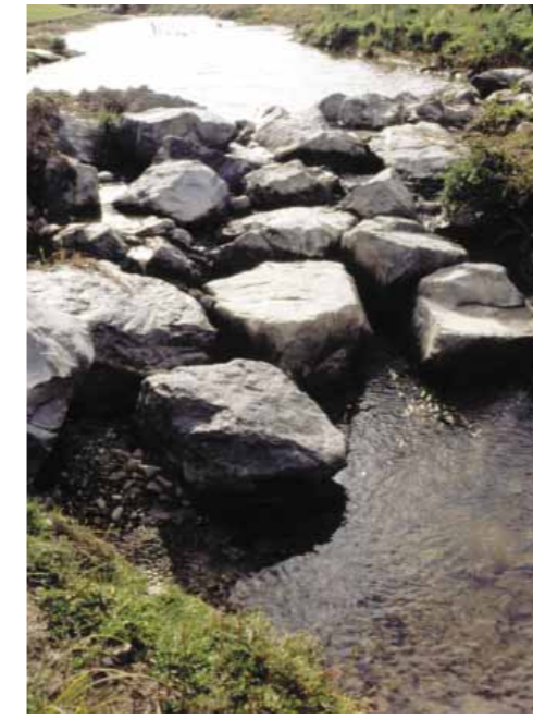
A rock ramp on a small stream is more fish-friendly than a vertical concrete weir
