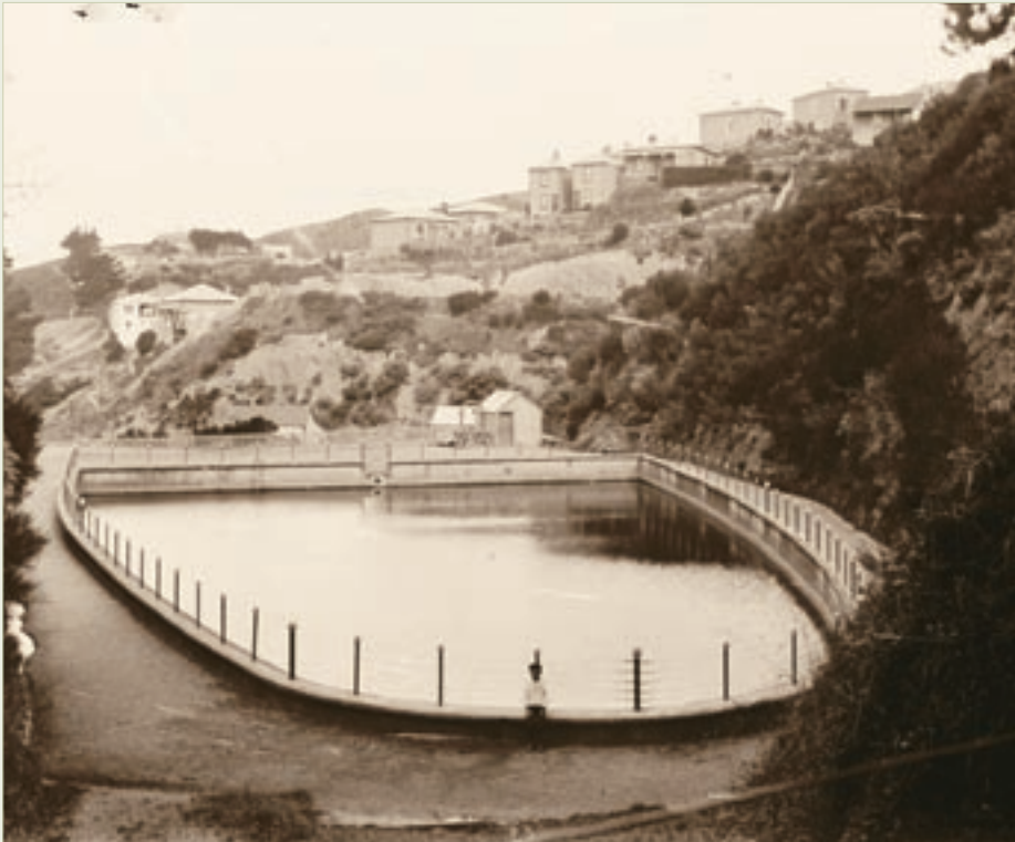
Polhill Gully reservoir, at the head of Aro Valley, circa 1900. This concrete distribution basin fed by the Kaiwharawhara Stream was the source of Wellington's first public water supply, in 1874. This distinction has often been credited to Karori's lower reservoir, which was not completed until 1878. (Alexander Turnbull Library, Wellington, NZ. Reference G-8021-1/2)
