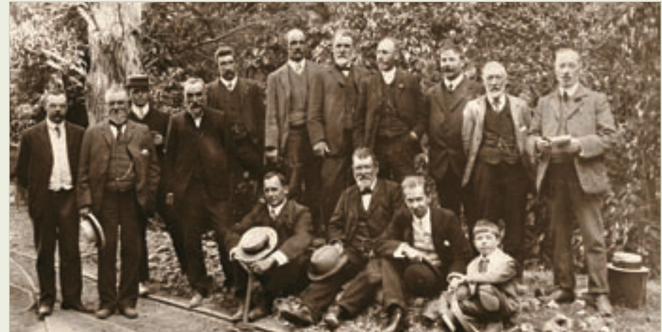
Contractors for the Karori upper dam, Mitchell & King, gather for the opening ceremony in 1908. (W F Tibbutt Collection, Alexander Turnbull Library, Wellington, NZ. Reference PAColl-0419)
