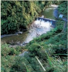
The water intake at Kaitoke on the Hutt River, seen here under construction (September 1952, left) and complete (above). Building the intake proved challenging, as it is situated in a narrow gorge that is subject to flash floods and the river could not be diverted away from the construction site.
