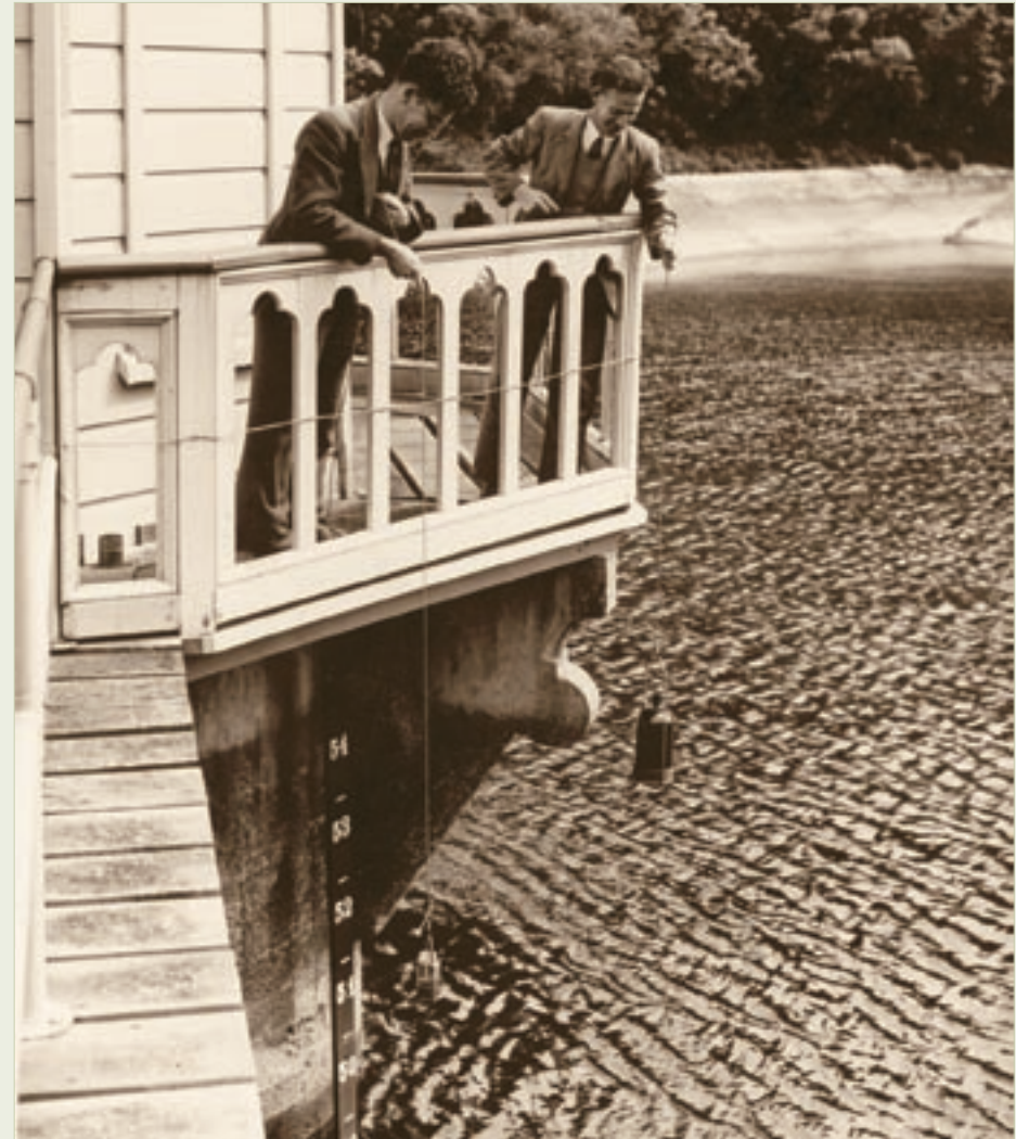
Wellington City Council Laboratory staff take water from Karori’s lower dam for testing, December 1952. Water from all sources was tested once a week. (New Zealand Free Lance Collection, Alexander Turnbull Library, Wellington, NZ. Reference F-92870-1/2)
