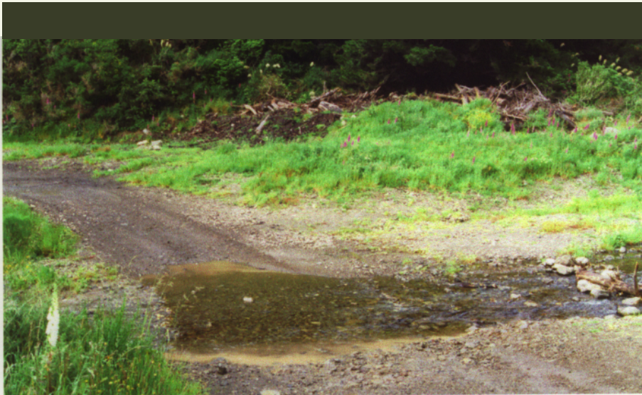
Logging debris adjacent to walkway
