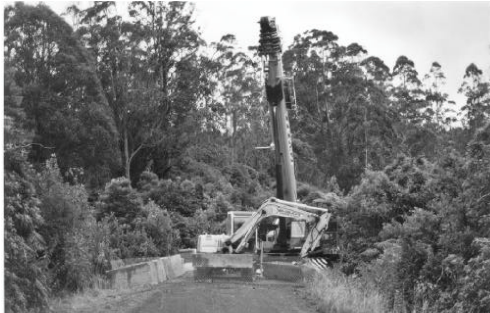
Crane for placing new pipes
