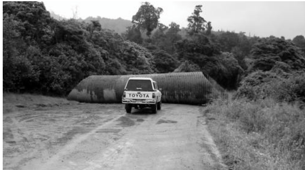
Old pipe removed
