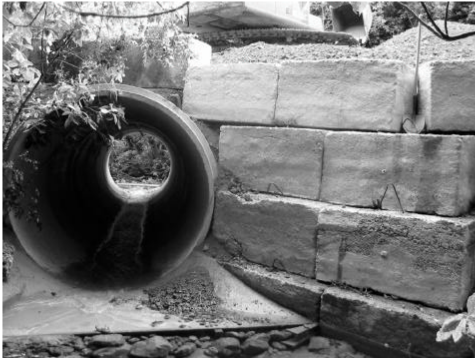
New pipes in place
