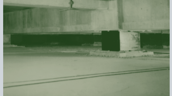
An example of a base isolator underneath Te Papa.
