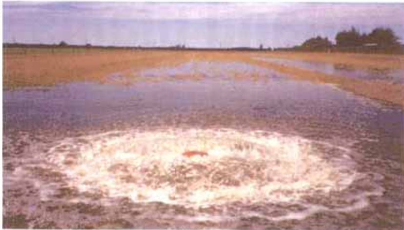
Bubble-up valves provide more precise discharging of treated wastewater for border strip irrigation.
