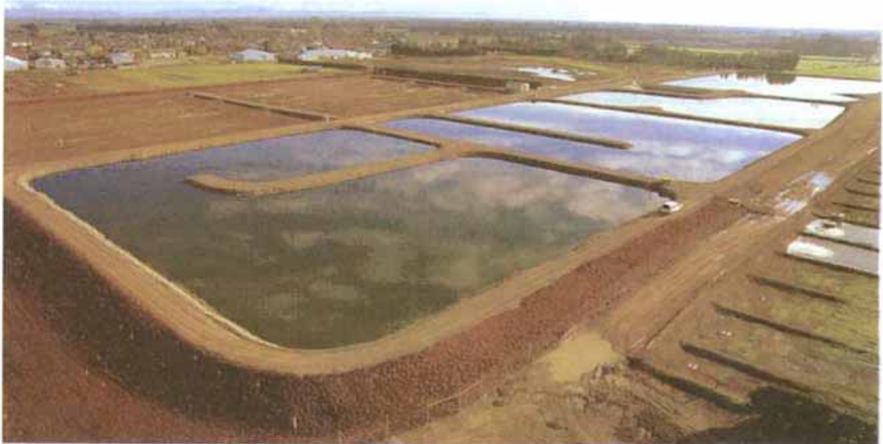
Aerial view of the treatment ponds - the original oxidation pond has been more than doubled in size and primary oxidation and maturation ponds have been added.
