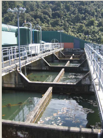
Flocculation tanks
