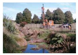
Construction of a new shallow monitoring borehole in Te Ore Ore as part of the Wairarapa groundwater investigation. This borehole, and ten others constructed across the valley, will support existing monitoring sites to help us understand the complex hydrogeological systems in the Wairarapa. At this particular monitoring site, we hope to further explore the link between the Te Ore Ore aguifer and the Poterau Spring seen in the foreground.
