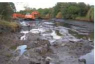
Contamination in this section of the Waiwhetu Stream in Lower Hutt was successfully cleaned up earlier this year. The stream was divided into two cells using sheet piles (left). The cells were then de-watered before the contaminated sediment was excavated from the upstream cell (right) and disposed of to landfill. The next stage of this project will be to remove the contaminants from the remainder of the stream.
