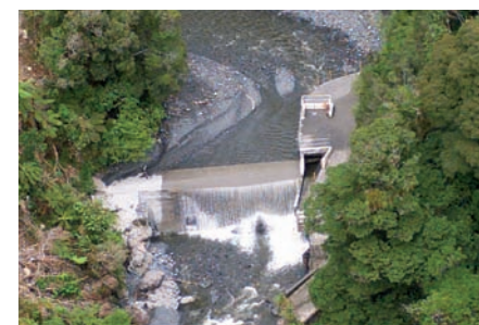
Orongorongo Weir: hydro generation is being considered
