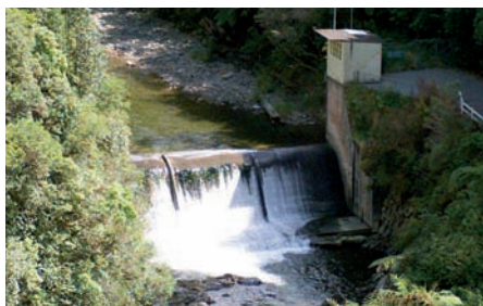
Kaitoke Weir: increased water take is being investigated
