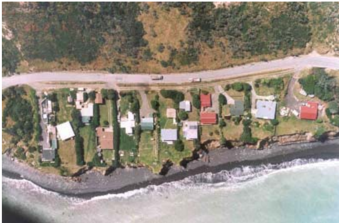
Figure 4.1. The typical nature of coastal land in eastern Palliser Bay. The top photograph shows the coastal road cut into the soft mudstone cliffs. An artificial boulder beach is currently being constructed to protect the road from disappearing completely. The bottom photograph, taken in February 2000, shows houses under threat at Whatarangi. Several buildings have been lost to the sea in this area. The amount of land lost in this area since 1996 is shown in Figure 8.
