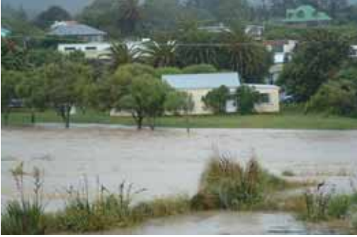
A severe rainstorm event on 7-8 January on the Kapiti Coast saw the Waikanae River flood properties in Otaihangā and threaten a number of homes.
