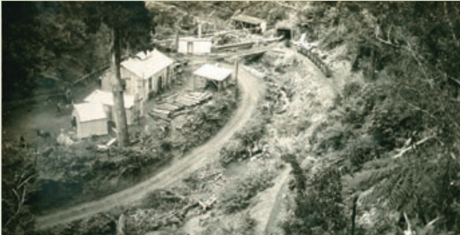
The western portal of the tunnel to link the Wainuiomata and Orongorongo water catchments, seen here during construction. The 3.2-kilometre tunnel took 28 months to complete, with tunnelling parties working from both ends.
