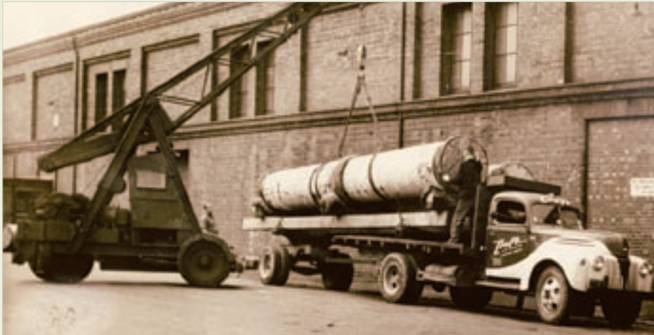
Stewart and Lloyds' steel pipes from Britain being loaded on a truck at Wellington wharf for delivery to Kaitoke, 1950
