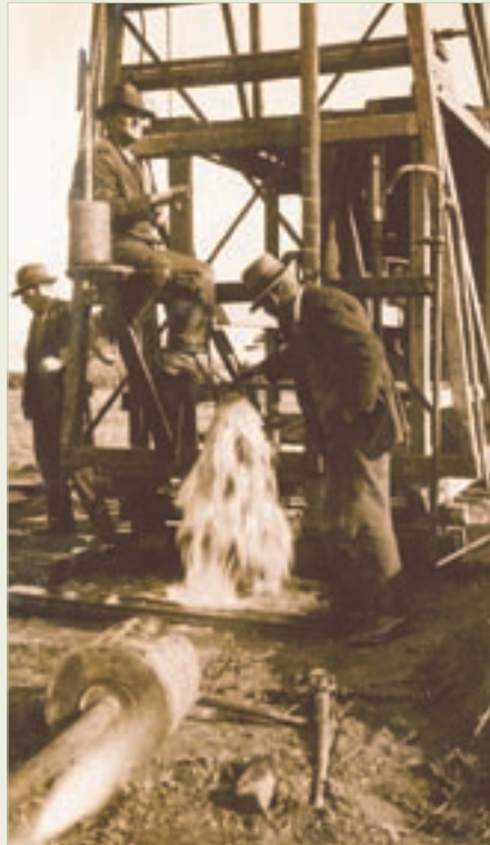
An exploratory bore at Gear Island. Artesian water had long been used in Petone when Wellington City tapped this source in the 1930s.
