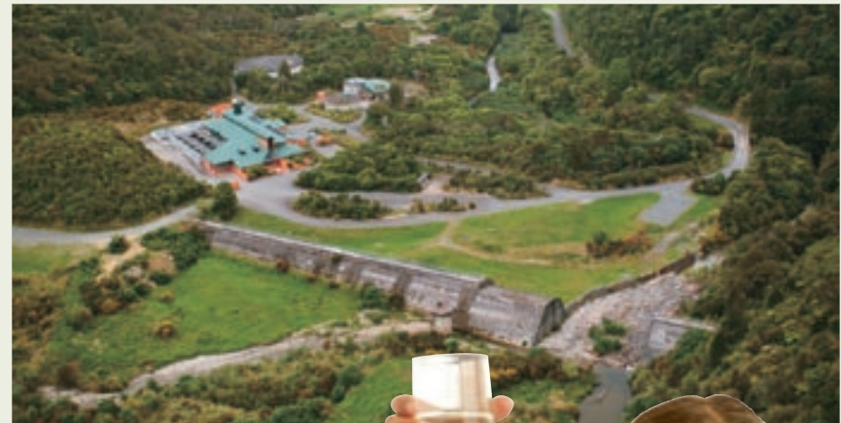
The Wainuiomata water treatment plant, with its state-of-the-art treatment process, was opened in 1993. The decommissioned Morton Dam can be seen in the foreground.
