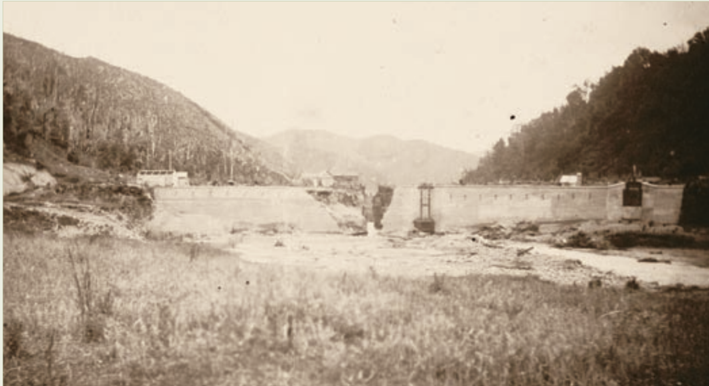
The first Wainuiomata dam in 1884, after it was breached by floodwaters. This failure and the subsequent controversy around its repair and the scheme's leakiness occupied Wellington's engineers and politicians for years to come. (Martin Album, Alexander Turnbull Library, Wellington, NZ. Reference PA1-f-036-13-2. Image cropped slightly)
