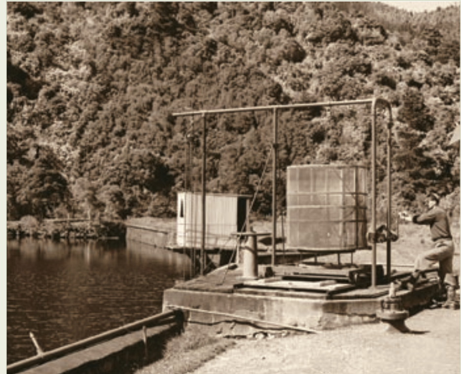
Cleaning the mesh filter at Wainuiomata lower dam, circa 1952. (New Zealand Free Lance Collection, Alexander Turnbull Library, Wellington, NZ. Reference PAColl-8983-27)
