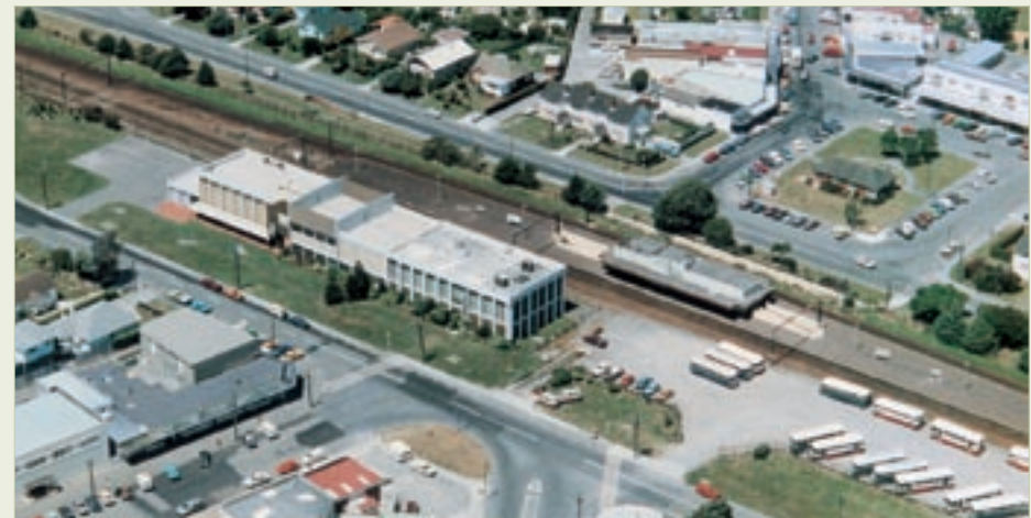
Waterloo water treatment plant and pumping station – next to the Waterloo railway station in Lower Hutt – became the main point of water abstraction from the Lower Hutt aquifer when opened in 1981 (photo December 1986).
