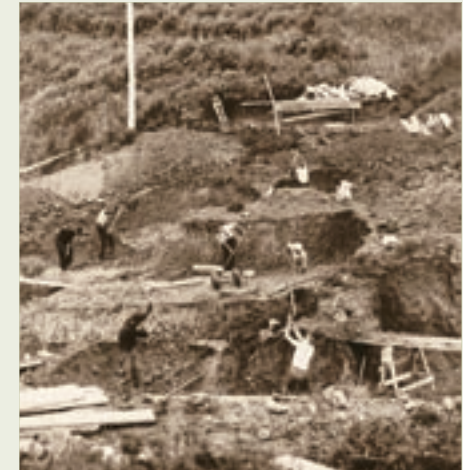
'Day' labourers excavating the site for the Eastbourne reservoir, located at Point Howard (circa 1930). (Alexander Turnbull Library, Wellington, NZ. Reference F-162468-1/2)
