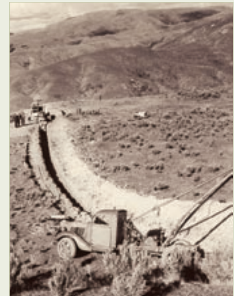
Laying of the Porirua branch line off the Kaitoke-to-Karori water main. (The Dominion Post, Wellington, NZ)
