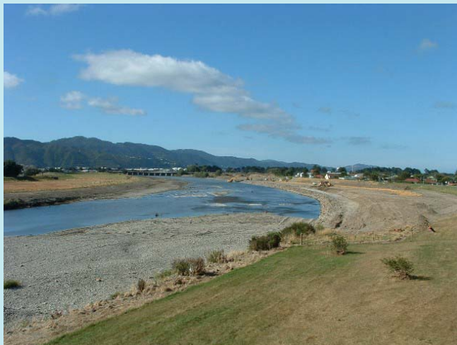
The Hutt River at Alicetown showing Stage One of the Eva to Ewen flood protection improvements (sourced from GW flood protection)
