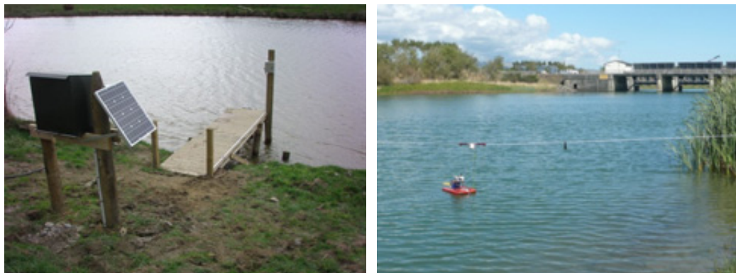
Figure 4.4: ADCP installation on the left bank of the lake outlet channel (left) and calibration gaugings (right - barrage gate is in the background)
