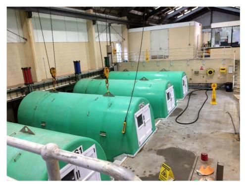
Figure 7: The Milliscreening Hall, with fibreglass covers over the screens to minimise  $H_2S/$  odour release
