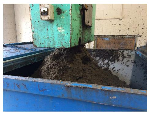
Figure 9: Dewatered sludge awaiting covering and transport for landfill disposal
