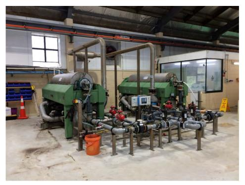
Figure 8: Sludge dewatering centrifuges
