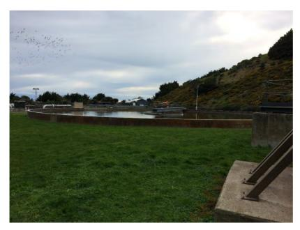
Figure 11: One of the three clarifiers used to settle remaining solids from the wastewater effluent prior to UV treatment and subsequent discharge via the ocean outfall
