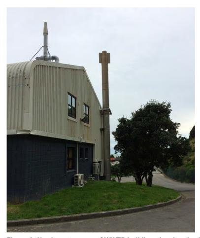
Figure 6: North-east corner of WWTP building showing the 10m discharge stack
