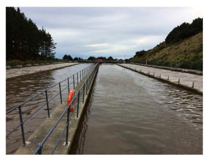
Figure 10: Aeration basin, with turbulence from active aeration being apparent in the side channels
