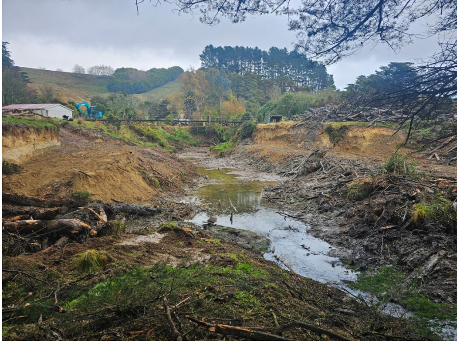
Figure 6: Kopuaranga River – Post blockage removal
