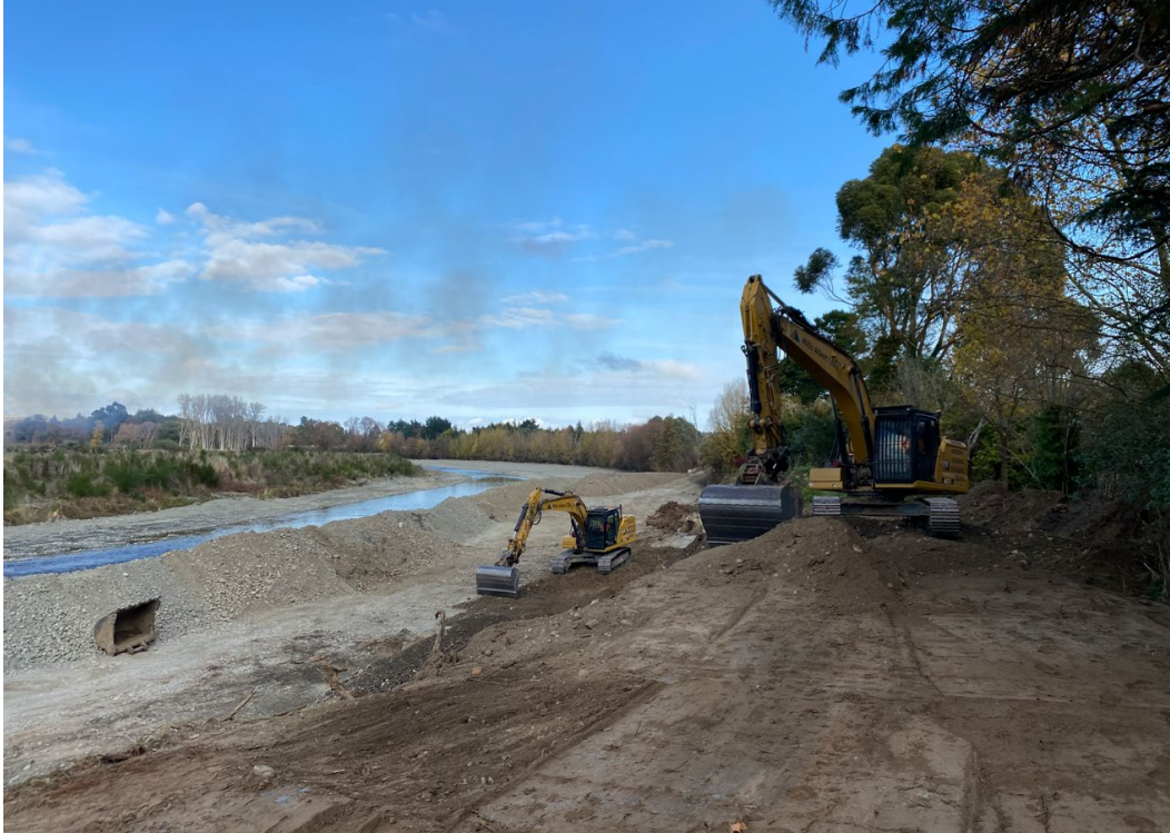
Figure 3: Stage two (Ruamāhanga River) – Shaping and profiling of the revetment batter
