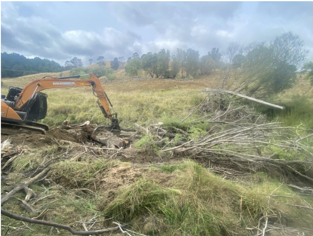
Figure 7: Whareama River – Blockage removal commenced
