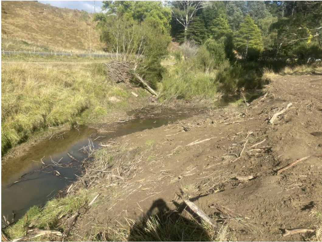
Figure 8: Whareama River – Post blockage removal
