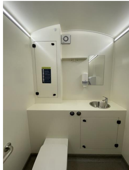
Image 4: Facility – installation in progress (Darlington Rd)
